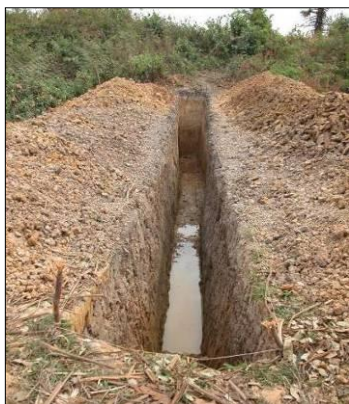
Fig. 19: Ground view of Northeastern Moat Trench
